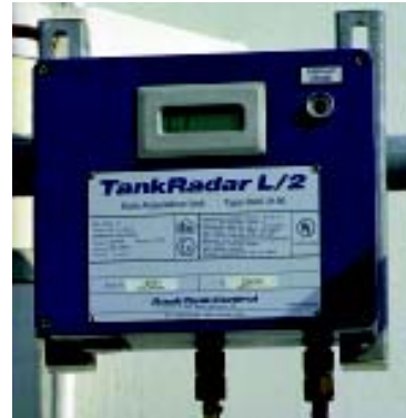
The Slave Data Acquisition Unit with Local Readout Display mounted at the foot of a tank.
