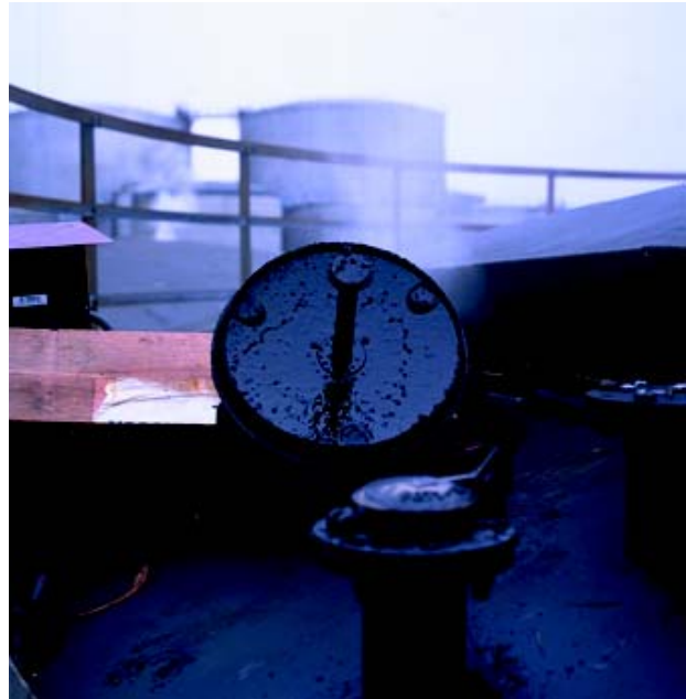
This gauge is still operating and gauging accurately despite the heavy contamination. The parabolic antenna has for several months been exposed to blown bitumen heated to over 220° C (430° F).
