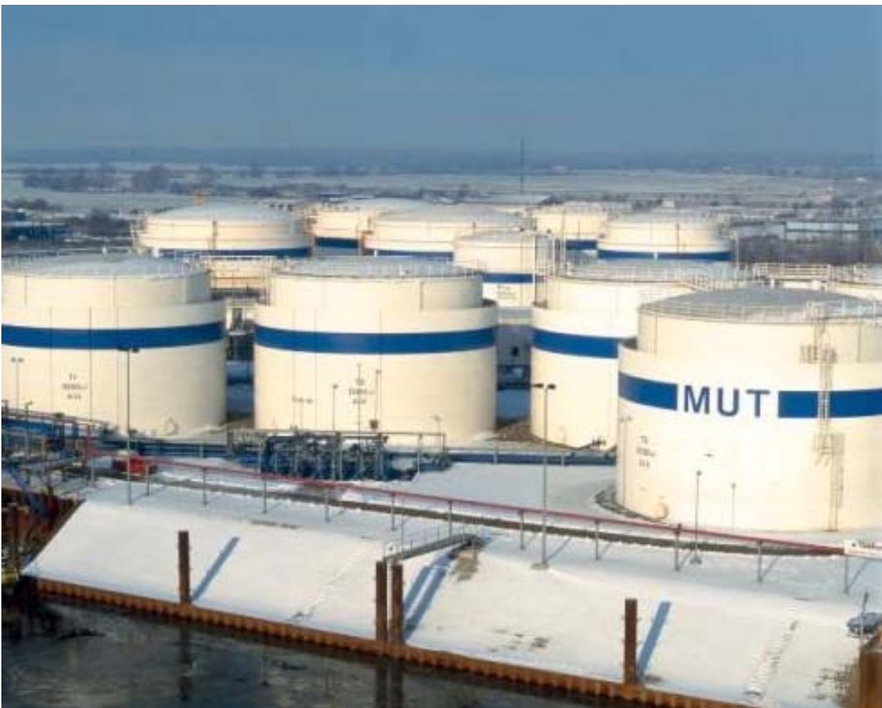
The FCU works as a data concentrator for a group of tanks ensuring fast data communication from the tanks to the control room.
